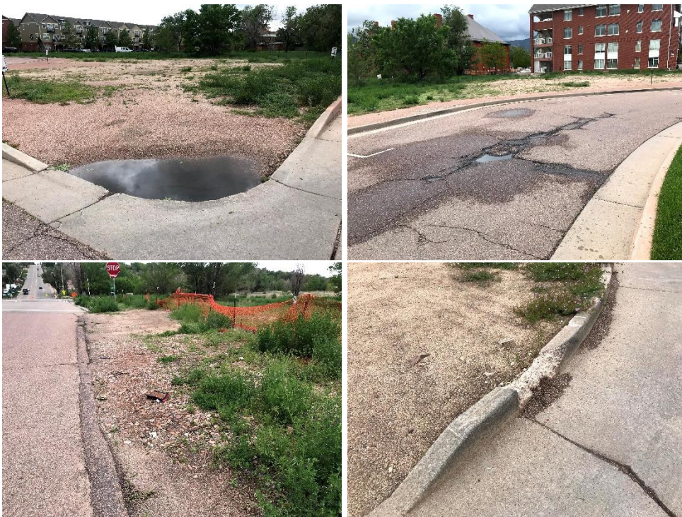
Figure 9. Deteriorated Pavement and Curbs and Missing Sidewalks
