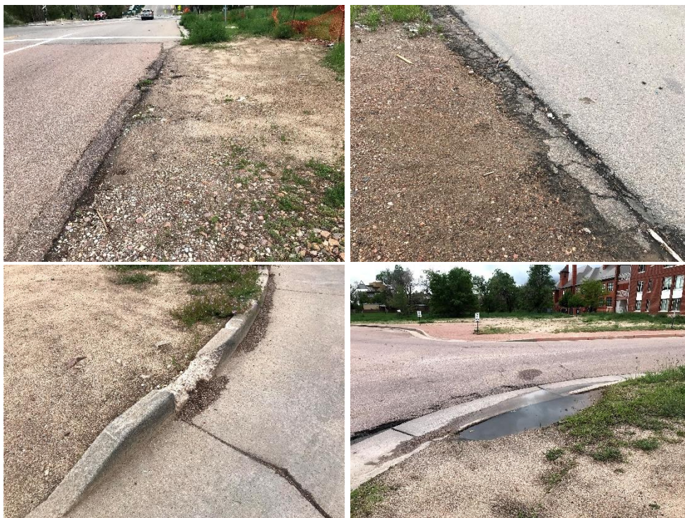
Figure 8. Deteriorated Curbs
