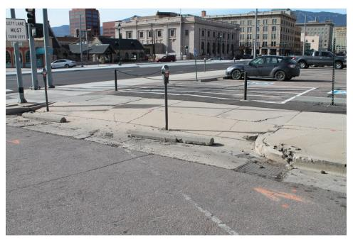
Figure 2-1 Poor vehicle access; substandard driveway definition; cracked or uneven pedestrian surfaces; insufficient grading; presence of trash and debris; potentially hazardous conditions; unsafe level changes; deteriorated pavement n ROW; deteriorated curb and gutter in ROW; deteriorated sidewalks in ROW; trip/fall hazard. (Photo 1)
