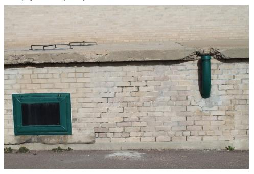
Figure 2-2 Deteriorated exterior walls; deteriorated exterior finishes; inadequate site maintenance. (Photo 5)
