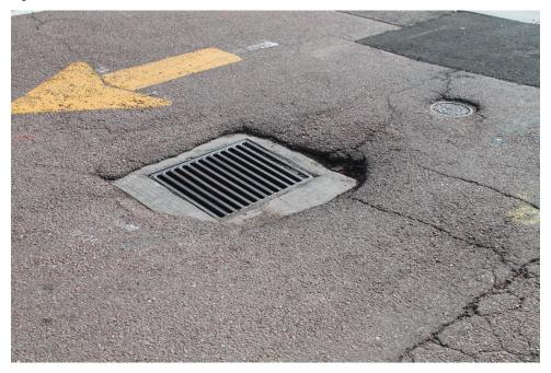
Figure 2-6 Poor drainage; unsafe level changes; deteriorated parking lot pavement; deteriorated surface drainage facilities; inadequate site maintenance; non-conformance to development regulations; unsafe level changes. (Photo 12)
