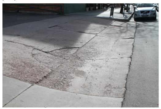
Figure 2-4 Poor vehicle access; substandard driveways; cracked or uneven pedestrian surfaces; presence of trash and debris; potentially hazardous conditions; unsafe level changes; deteriorated curb and gutter; deteriorated sidewalks; deteriorated surface drainage facilities; inadequate site maintenance; non-conformance with development regulations. (Photo 17)
