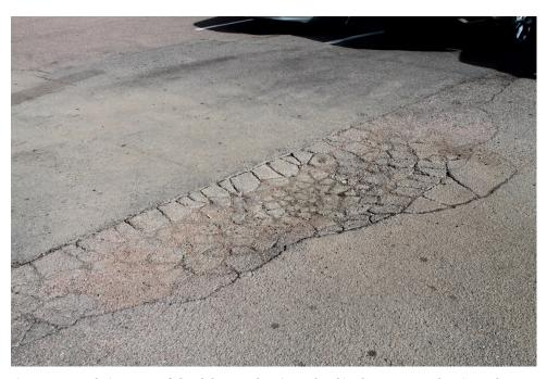
Figure 2-5 Poor drainage; unsafe level changes; deteriorated parking lot pavement; deteriorated surface drainage facilities; inadequate site maintenance; non-conformance with development regulations. (Photo 22)
