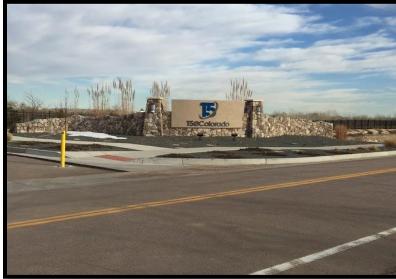
West Side Entrance
