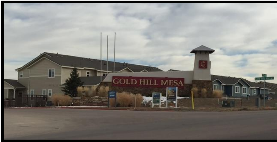
Twenty-first Street Entrance
