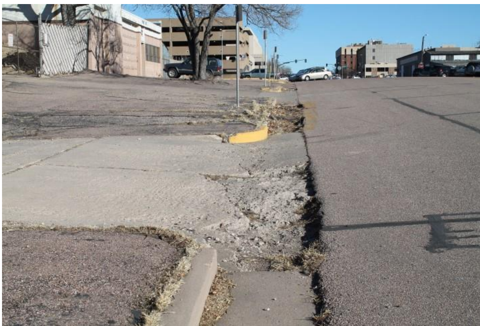
Figure 2-5 Presence of trash and debris, substandard driveway/curb cuts, cracked and uneven surfaces, unsafe level changes, deteriorated curb and gutter, inadequate and deteriorated sidewalk, inadequate site maintenance, non-conformance to development regulations (Photo B-11)
