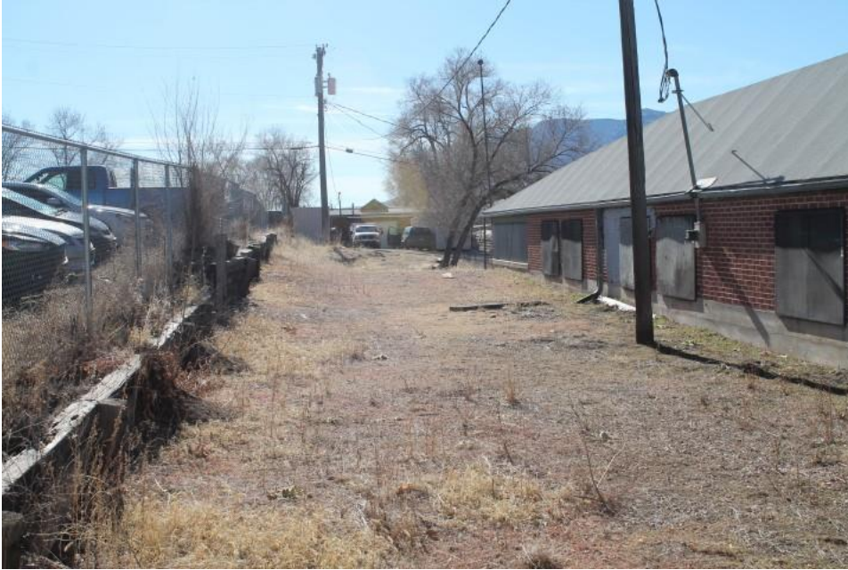
Figure 2-10 Presence of trash and debris, vagrants/graffiti/vandalism (Photo D-5)
